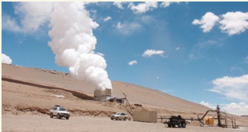
Conducting a well testing
