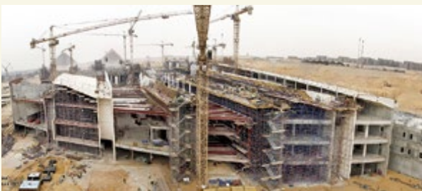
Construction site of the new museum with pyramids in the background.
