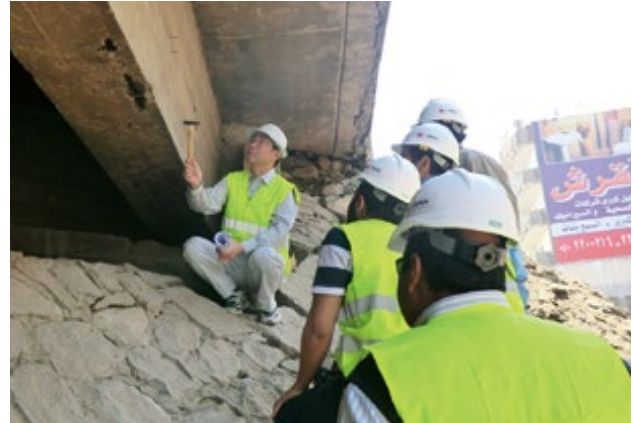
Egyptian engineers receiving guidance on bridge inspection methods (The Project for Improvement of the Bridges Management Capacity)
