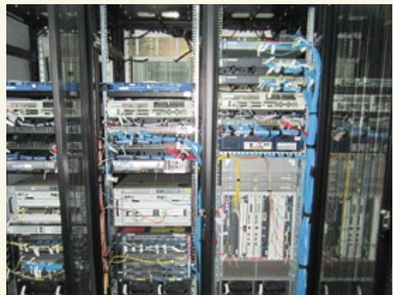
Communication equipment deployed in this project contributed to improving the communication environment in Myanmar.
