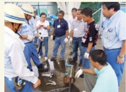
A scene from plumbing training conducted at the Water Works Bureau of Yokohama City
