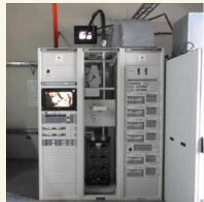
EWBS digital transmission equipment (Photo: Yachiyo Engineering Co., Ltd.)
