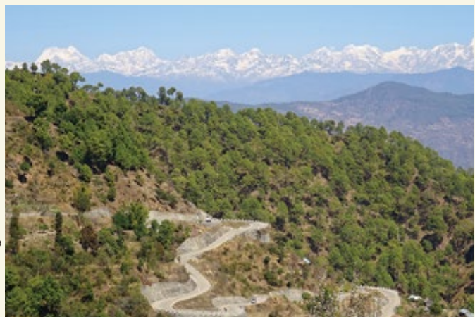
The Sindhuli Road meanders through the Mahabharat Range, with the Himalayas in the background. (Photo: Nippon Koei Co., Ltd.)
