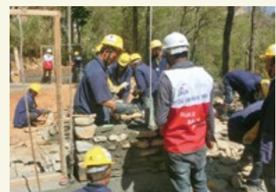
A construction expert providing guidance on how to make buildings more quake-resistant.
