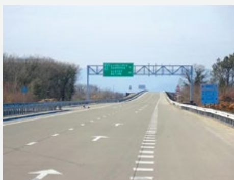
The section is already open and operating. JICA is committed to more assistance toward the completion of the entire East-West Highway.
