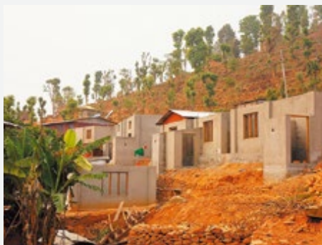
Houses being rebuilt by home-builders who received JICA training
