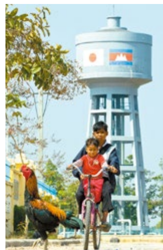
Cambodia: A water tower managed by Siem Reap Water Supply Authority under the Project on Capacity Building for Water Supply System [photo by Kenshiro Imamura]
