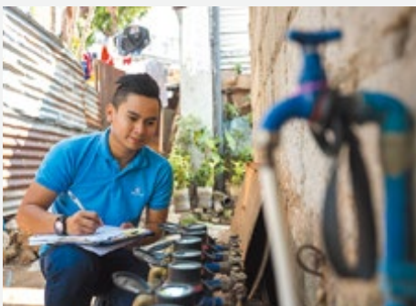
An employee checking water meters [photo: Maynilad Water Services, Inc.]
