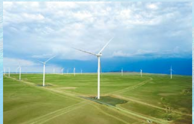
Mongolia: JICA co-financed the Tsetsii Wind Farm, a private-led project, with the European Bank for Reconstruction and Development under the Private-Sector Investment Finance program. The project is the second renewable energy project in the country.
