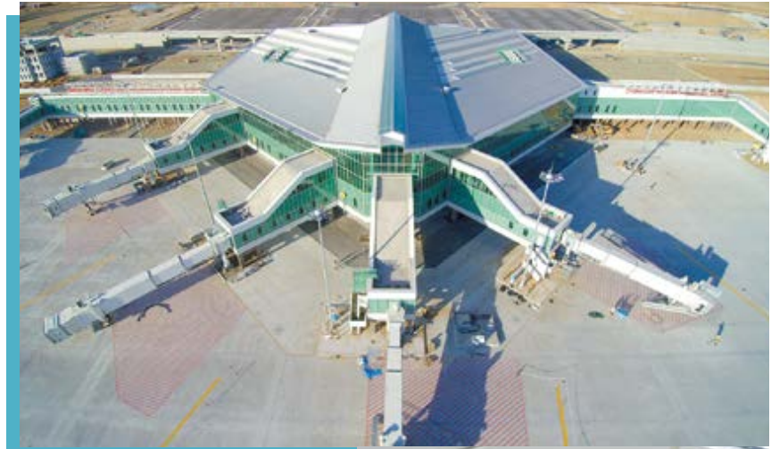
A complete view of the newly completed Chinggis Khaan International Airport, Mongolia's first private-operated airport (above)
