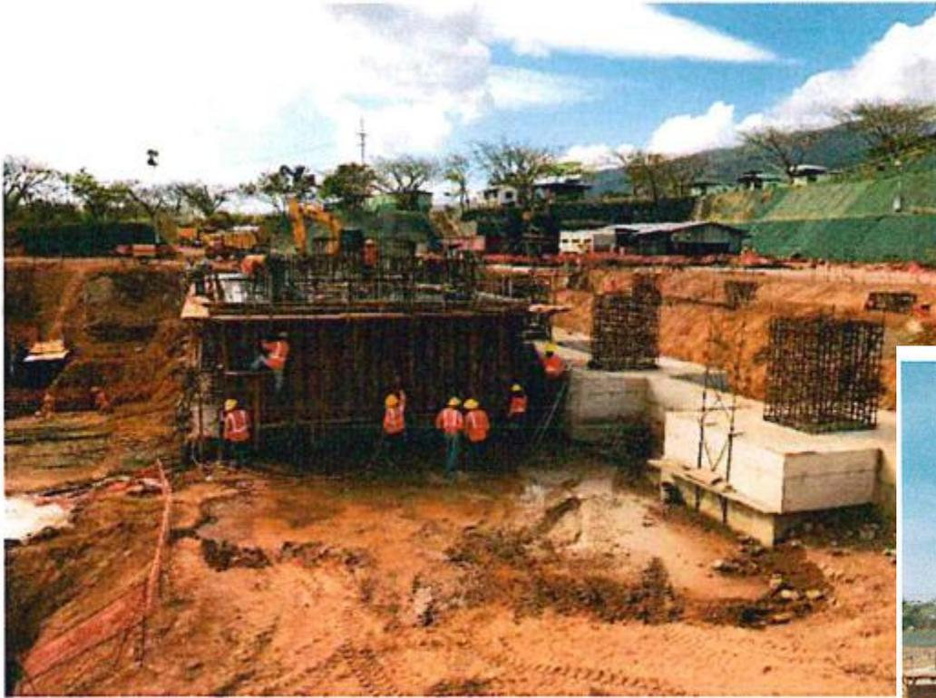
Picture 1: turbo-generator foundation (03-14-2017).
