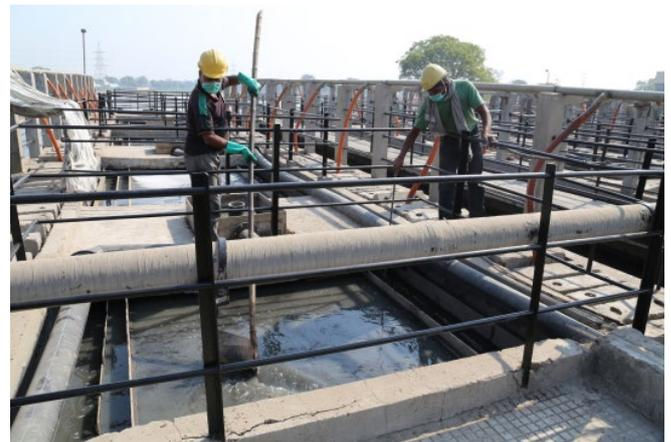
Cleaning of Impurities from Grid at Agra Water Treatment Plant
