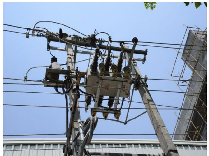
Load Break Switch (LBS) – automatically Isolate Faulted Sections of Electrical Distribution Systems at Bangalore District Upgradation Project
