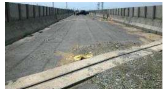
Access Road to Kamarajar Port (Ennore Port)
