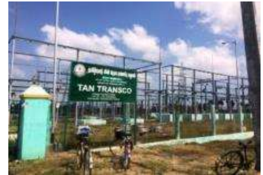
110kV Substation at OneHub Chennai Industrial Park
