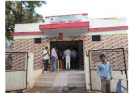
A community toilet installed under JICA ODA loan project
