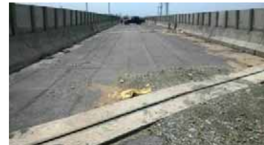
Access Road to Kamarajar Port
