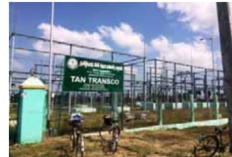
110kV Substation at OneHub Chennai Industrial Park
