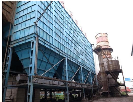
Electric dust collector installed into Steel Plant
