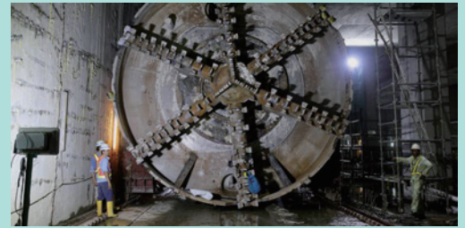
3: Shield excavator
