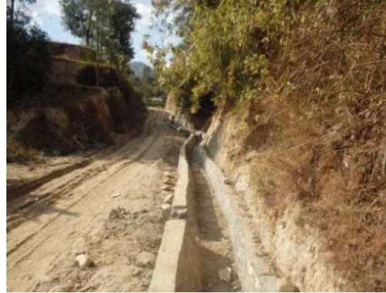
Bhotechaur Road & Irrigation Facilities
