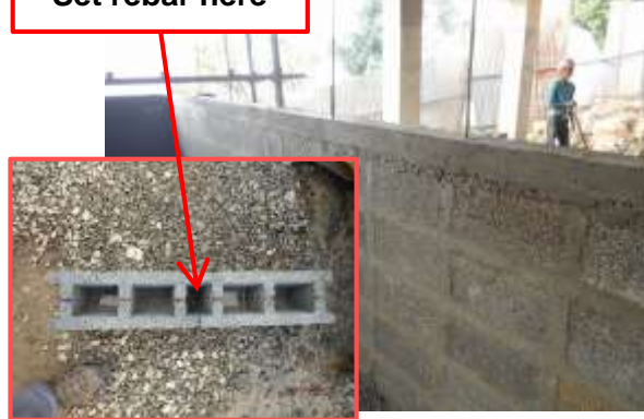
Rebar in hollow block walls
