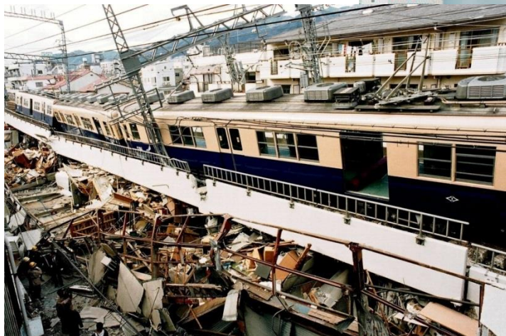
Damaged railway track
