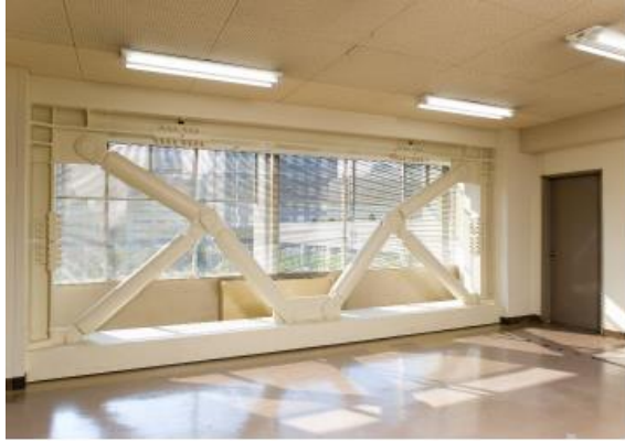
Seismic Brace with vibration damper inserted.
