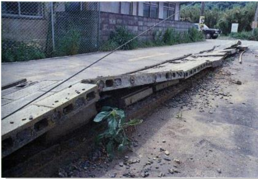
Crashed concrete block wall school children crushed to death
