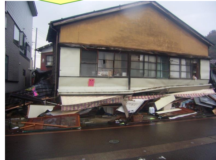
Collapse of houses built before 1981
