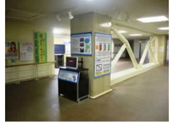
Seismic Brace & Seismometer installed on ground floor hall.
