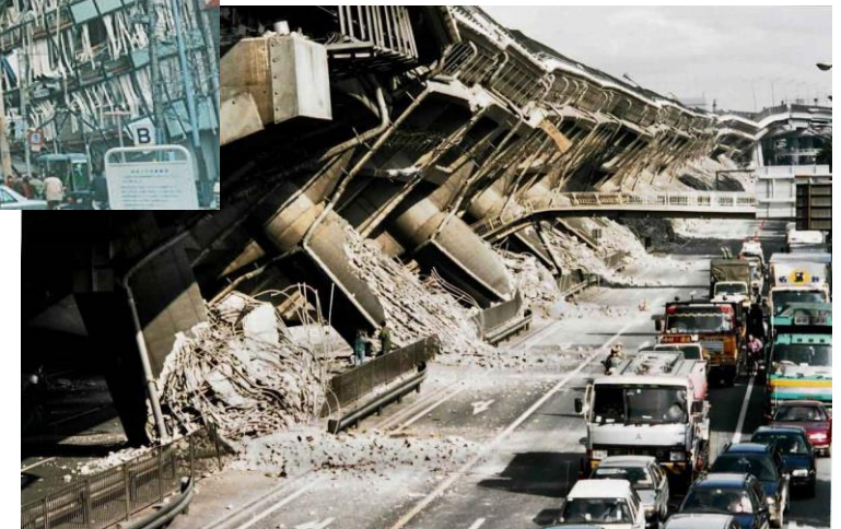
Collapsed viaducts of an expressway
