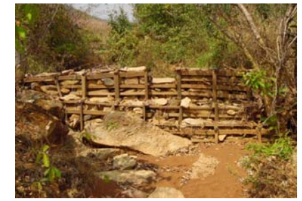
Constructing small check dams
