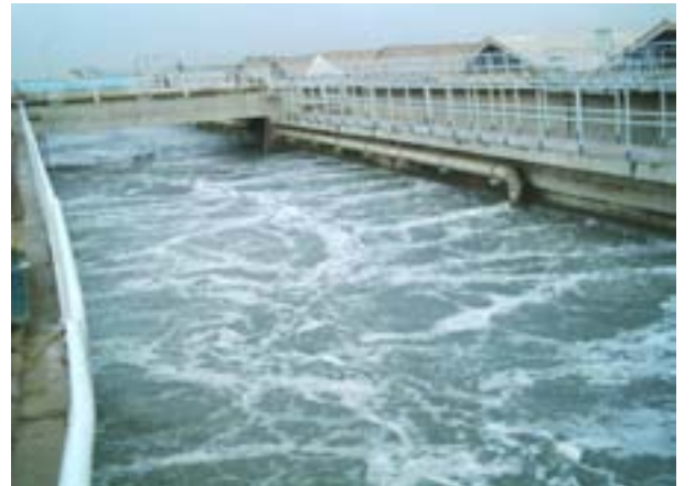
Grease Removal Tank
