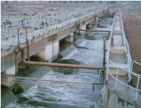
Grit Removal Channel
