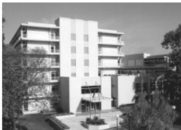
Photo 1 New BMH ward constructed as a Japanese government's Grant Aid Cooperation project
