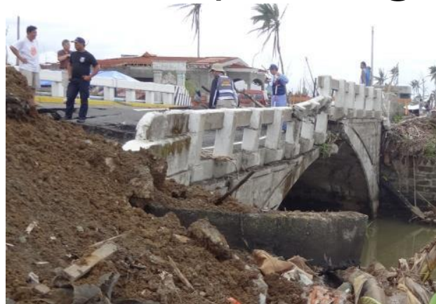
Damaged bridge by tidal wave
