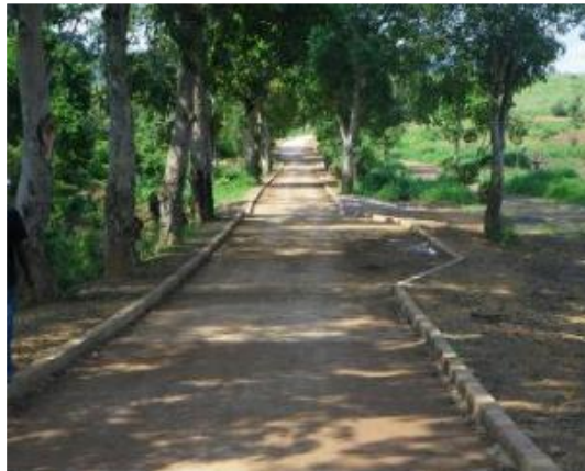
Community road after rehabilitation
