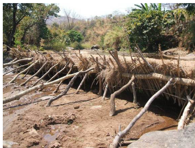
Temporary irrigation made of wooden poles and grass
