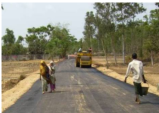
Rural road being constructed by LGED Photo: LGED
