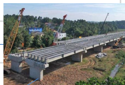
Construction of Outer Circular Highway Project Phase III from Keralalapitiya to Kadawatha
