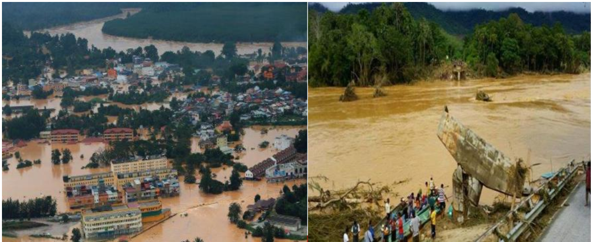
Figure 5: Situation of flood in Kelantan 2014 flood where major infrastructure such as bridge collapsed during the flood.
