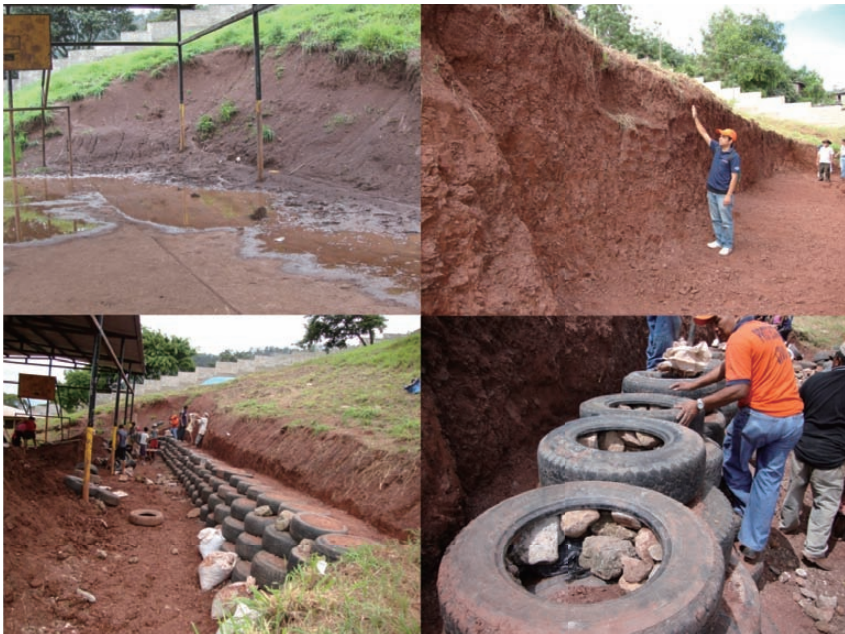
Figure 8: Construction of a Used-tire Retaining Wall to Avoid Land Slides in Honduras
