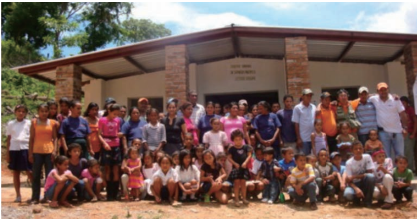
Figure 14: Centro Albergue (a Community Shelter House) in the Metapalos Arriba Community in Cholteca, Honduras.
