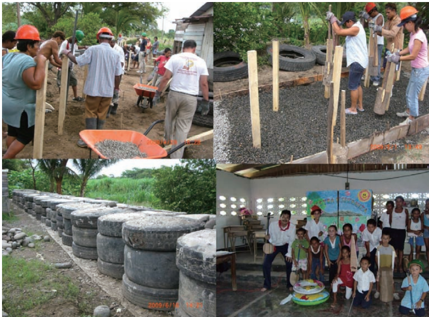
Figure 7: Construction of Used-tire Dyke in Costa Rica
