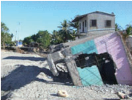
(Above) House destroyed by Hurricane Ida in Las Ojas community in November 2009
