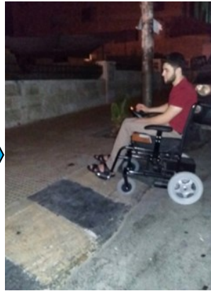
After : Ramp was installed
