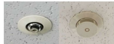
Left: Sprinkler Right: Heat and Smoke Sensor
