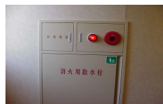
Left: Emergency Telephone Right: Alarm Button Bottom: Fire Hose
