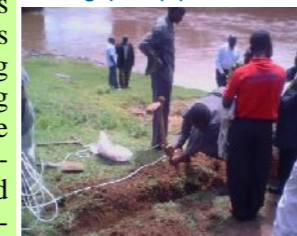
WRUA members dig trench to lay in cabling pipes that links the gadget at the river and alarm at observer's house
