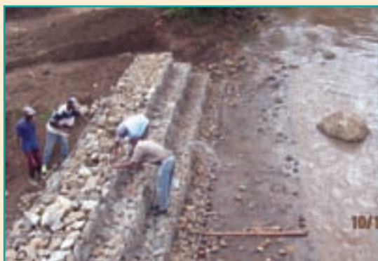
Community members constructing gabions for riverbank protection at Chil Chila.
