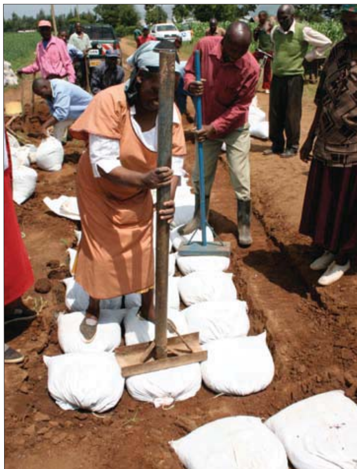
Farmers repairing a rural road at Kabatini using 'Do-nou' technology.
