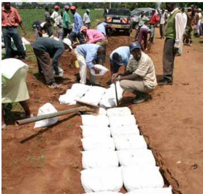
Farmers at Bahati, Nakuru repair the road to their farms using 'Do nou' technology.
