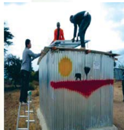
Installation of Charging System in a school.
