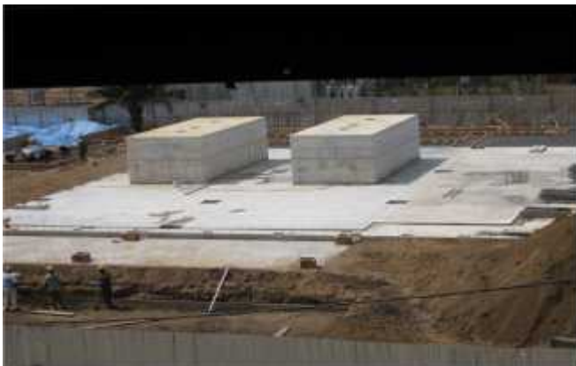
Completion of foundation for the Powerhouse
