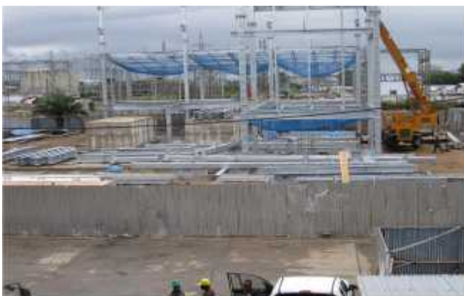
Commencement of steel structure works for the Powerhouse
