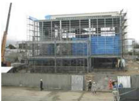
Completion of structural steel works
