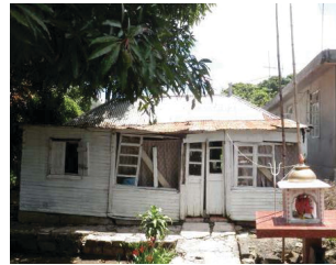
Deformation of the house
