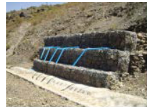
Installation of drainage
