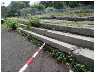
Deformation in the steps
