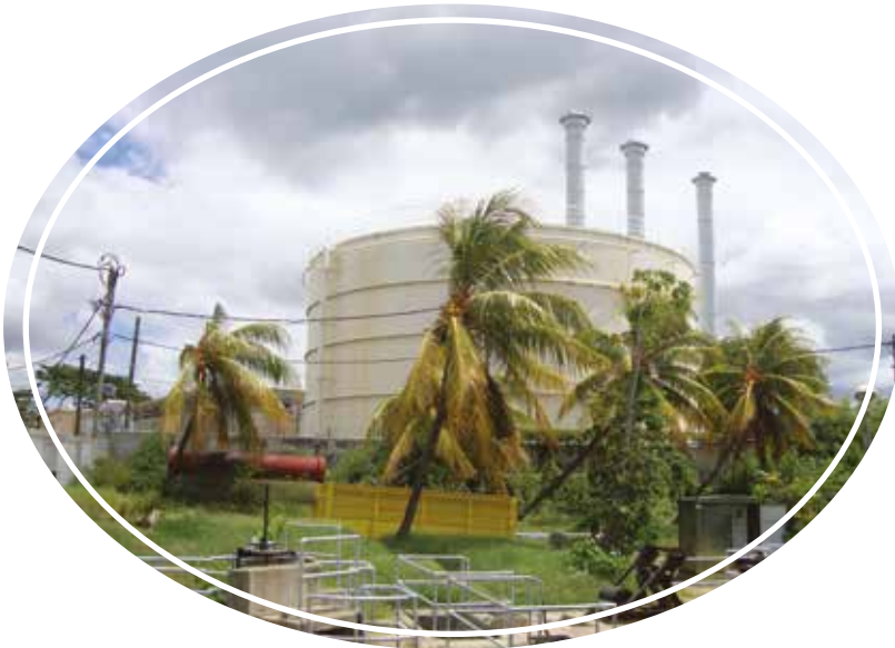
Grand Baie Treatment Plant
