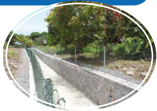
Landslide countermeasure work at Chitrakoot
