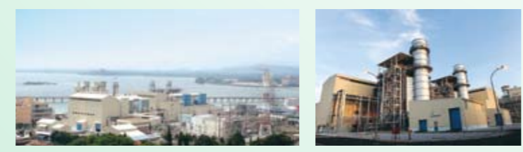
Port Dickson Power Plant
