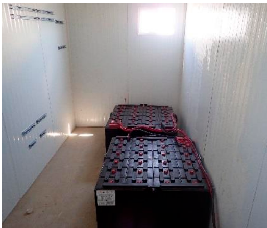
(a) Battery bank
