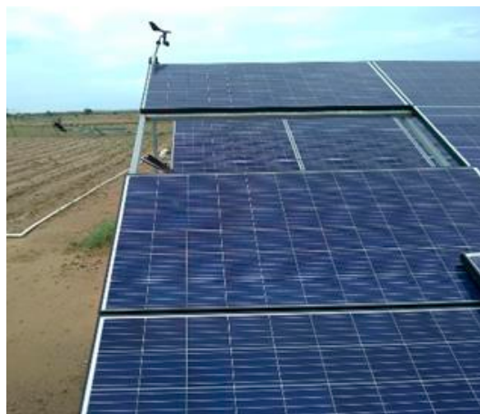
Photo.5 Damage of PV array by hurricane
