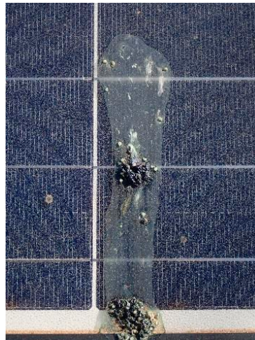
Photo.7 Soiling on PV panel
