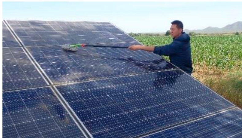
Photo.1 Cleaning surface of PV arrays
