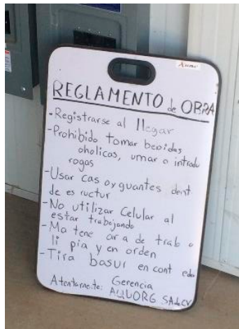
Photo.4 Sign and warning for electrical equipment
