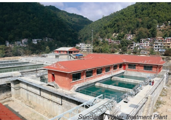
Sundarjal Water Treatment Plant
