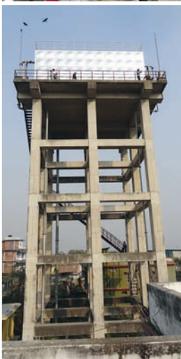
Rehabilitation of water tank in Dhulabari, Jhapa.
