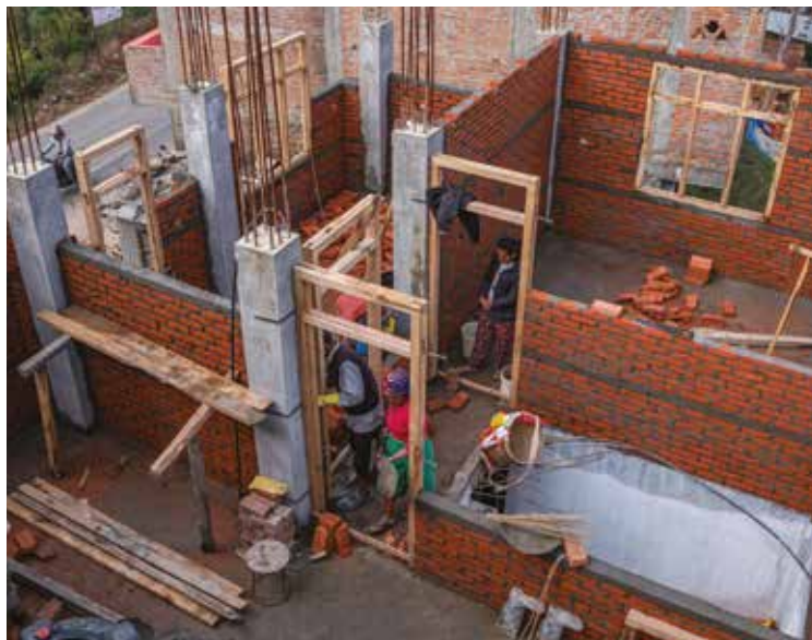
House under construction in Sanghachowk, Sindhupalchowk
