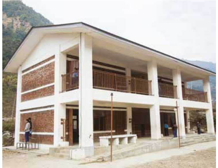
Earthquake resistant school built by JICA
