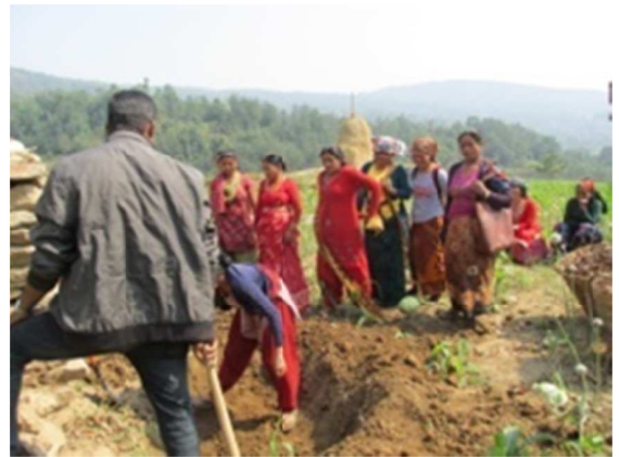
Fig. No. 12.1.2 Taking out soil from pit
