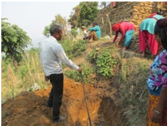
Fig. No. 12.1.3 Pit ready for putting compost making materials
