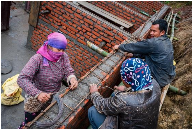
Earthquake resilient house is being constructed by house owners.
