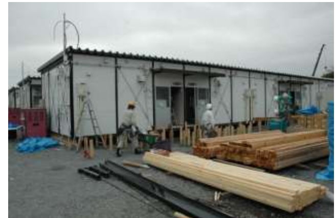
Construction of temporary housing
