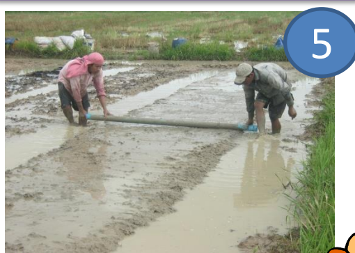
Leveling surface of bed
