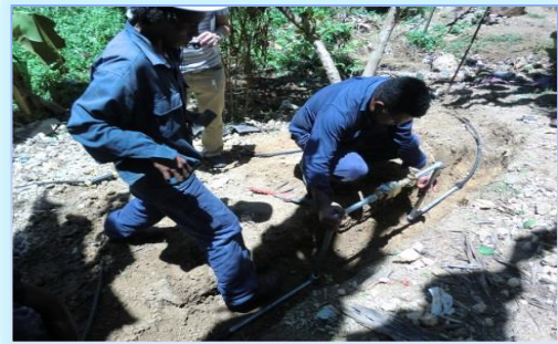
Photo-4 Installation work of water
