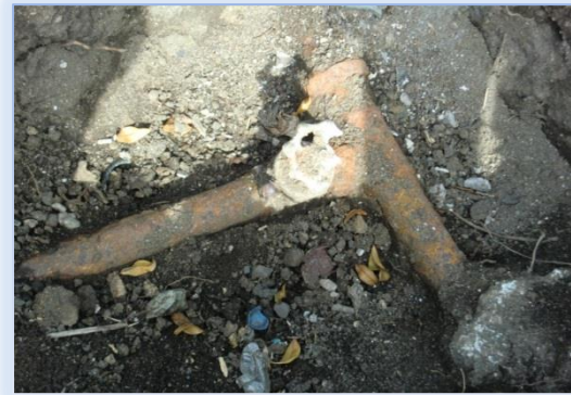
Photo-7 Over 60 years old pipes after installation
