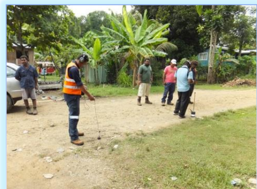
Photo-5 Identification of leakage points by using leak detection equipment
